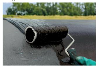
The new **FORTIDE**® Epoxy coatings guarantee the 100% Made in Germany quality from industry leader DENSO. They are suitable for the rehabilitation of pipelines, as a whole pipe coating or for welded joints and complex geometries. The products are characterised by an outstanding coating hardness and exceptional indentation strength. All **FORTIDE**® products are **free of VOC & isocyanates** and fully comply with **ISO 21809-3**. **denso-group.com**
