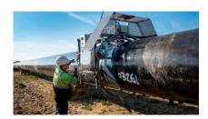
**DEKOMAT®-11** is a portable automated wrapping machine that is powered by a petrol engine. **DEKOMAT®-11** is ideally suited for use in pipeline section rehabilitation and field-joint coating in new construction work. With its two roll holders, it offers the option of processing multilayer tape systems in a single work step.
