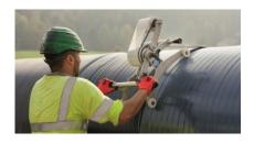
**DEKOMAT®-KGR Junior** has been designed for processing larger roll lengths. **DEKOMAT®-KGR Junior** is the perfect choice for tackling the challenges of larger nominal pipe sizes. With the optionally available accessories, wrapping is possible for pipes with nominal sizes of DN 2000 and over.
