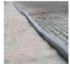
Simple insertion, overhang by 5mm on rolled asphalt
