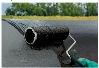
The new **FORTIDE**® Epoxy coatings guarantee the 100% Made in Germany quality from industry leader DENSO. They are suitable for the rehabilitation of pipelines, as a whole pipe coating or for welded joints and complex geometries. The products are characterised by an outstanding coating hardness and exceptional indentation strength. All **FORTIDE**® products are **free of VOC & isocyanates** and fully comply with **ISO 21809-3**. **denso-group.com**
