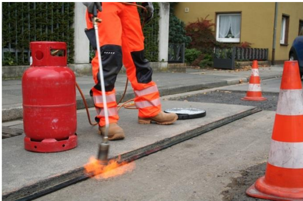
TOK®-Band A applied in seconds
