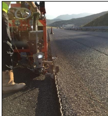
Fig. 2: Joint installation using the TOKOMAT® process
