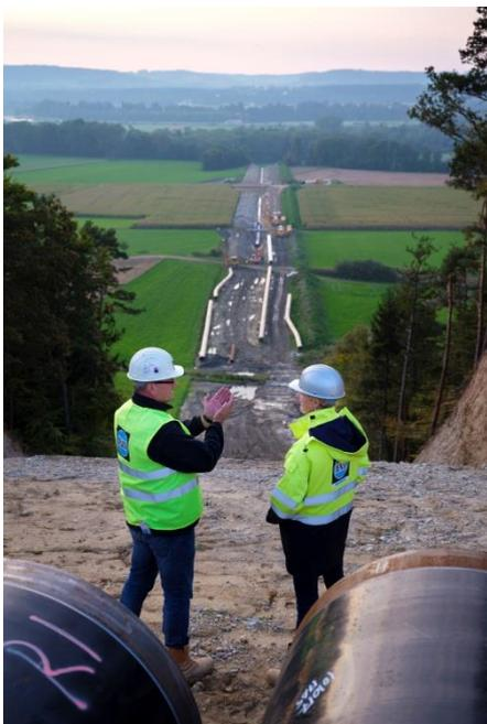
Image caption: Steep slope at the installation site of the high-pressure gas line *MONACO* in Upper Bavaria
