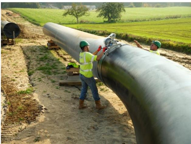
Image caption: Fast and precise application of DENSOLEN<sup>®</sup>-N60/-S20
