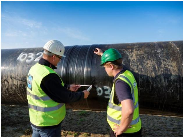
Image caption: Corrosion prevention for approximately 3,000 welded seams
