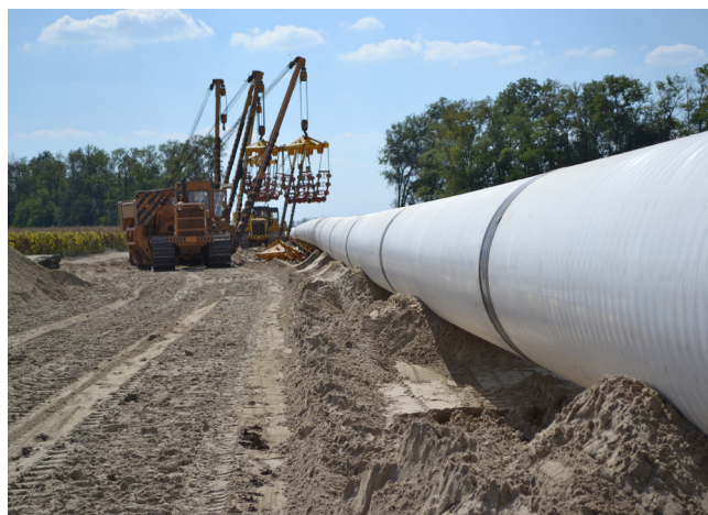
Figure 3. A pipeline with welding areas protected by DENSOLID-HDD.
