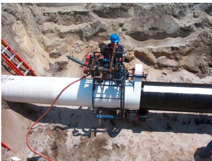
Seal For Life Industries: Pipeline CAT rehabilitation.
