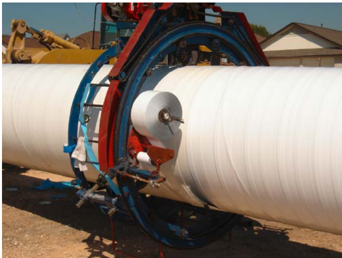
Seal For Life Industries: Pipeline CAT coating.
