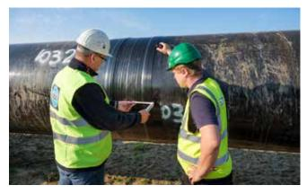
Figure 5. Quality inspection of the overlap width.
