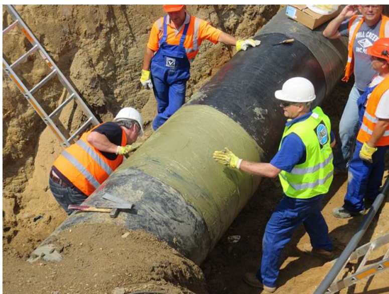
Figure 1. Application of DENSO-AO primer.
