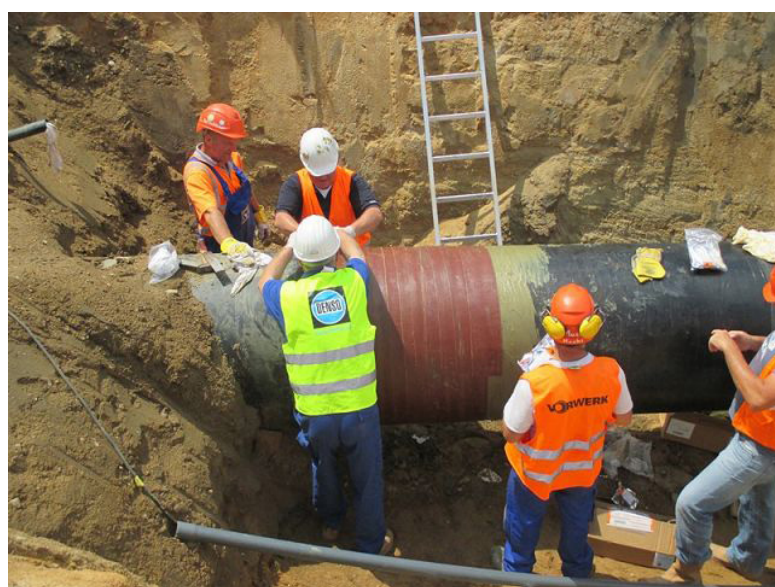
Figure 2. Application of DENSO-MT petrolatum tape.
